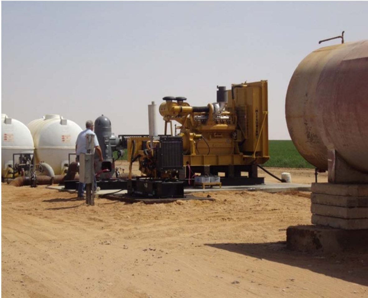
Fig. 4 Existing pumps Q = 340 \text{ m}^3/\text{h} , H = 330 \text{ m} , P = 725 \text{ HP}
